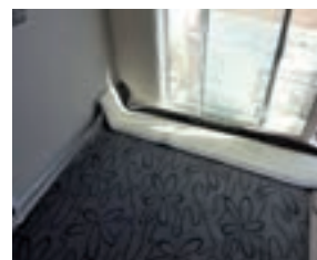
Laying the carpet
