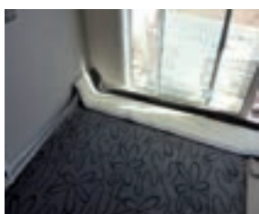
Implantation de la moquette Laying the carpet
