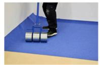
Roll the sheet or press into the adhesive with a rubbing board or glider within the open time of the adhesive.
